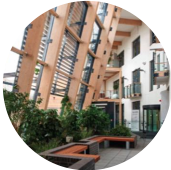
Hempcrete in University of Bradford's Business Center [2]
