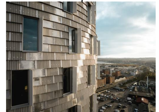
TRÆ – an example of End-Of-Life wind turbine blades incorporated into architectural design of a building.
