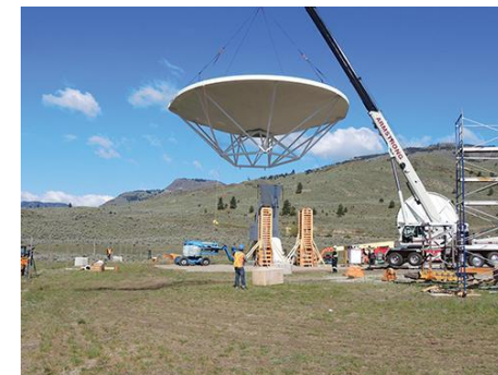
Installing disk on base
